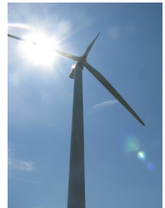
Windmill on site.
